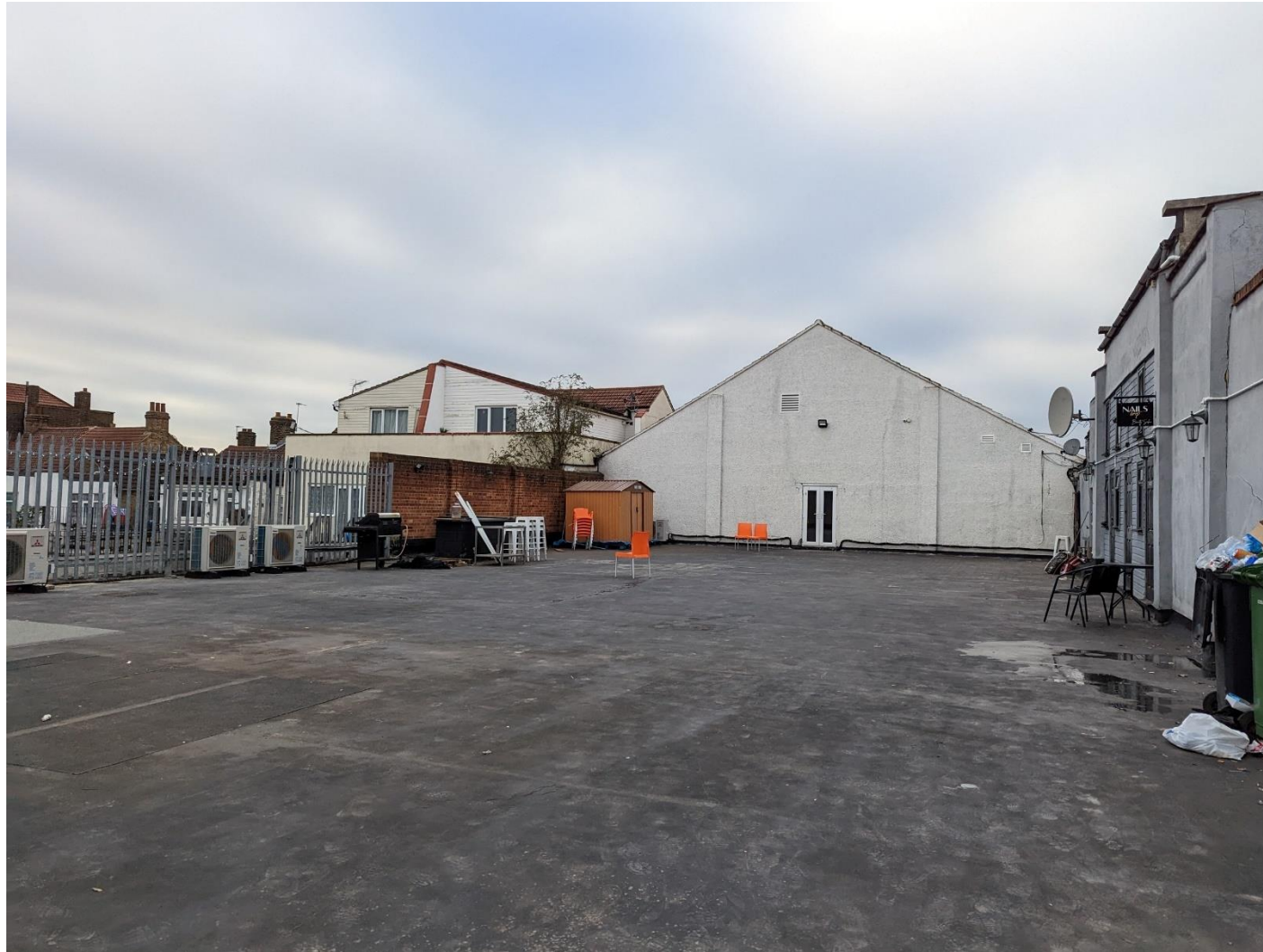
Photo 6 Flat roof (first floor level), facing west
